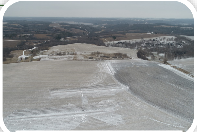
A series of three basins installed to reduce soil erosion in the Little Cannon River Watershed in Goodhue County
